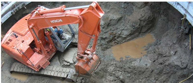
Excavation is proceeding on the Custer Avenue Storage and Dechlorination Facility.
