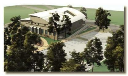
This parking lot features Pervious concrete with a retention pond below. The lot is maintenance free and no rain water leaves the site.
