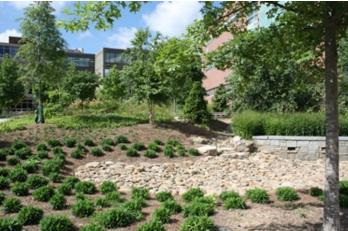
Klaus' bioretention areas accept building's roof runoff and first flush into two underground cisterns, with a combined volume of 174,149 gallons. The bioretention area of the site used 350 cu yd of engineered soil, comprised of 40% clay topsoil, 20% sand, 20% ERTH food compost and 20% HydRocks. Manufactured by Big River Industries, HydRocks is an expanded clay aggregate product, manufactured through a rotary kiln process in which selectively mined clay is fired at 2,000°F.
