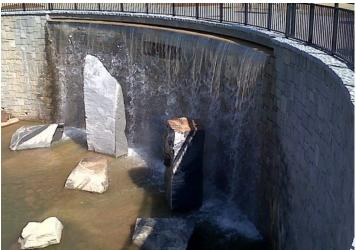
The Old Fourth Ward Stormwater detention pond has enough capacity to hold a 500 year storm event. Rain water recedes to Highland Ave. combined sewer trunk. In the case that the trunk fills, it has been retrofitted to prevent flow back into the basin.
