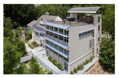
Southface's 2,000 sq ft green roof includes a 6.4 KW photovoltaic array and reflective roof pavers. A 1,750-gallon cistern collects rainwater for toilet flushing, rooftop irrigation, and an evaporative mesh cooling system. It is wrapped in a wooden vat salvaged from an abandoned winery in South Atlanta. Tours of this facility are available by appointment, (404) 872-3549.
