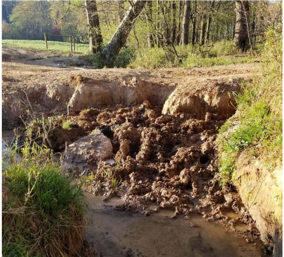
**Before:** A failed and undersized 24-inch round culvert that did not exclude livestock.
