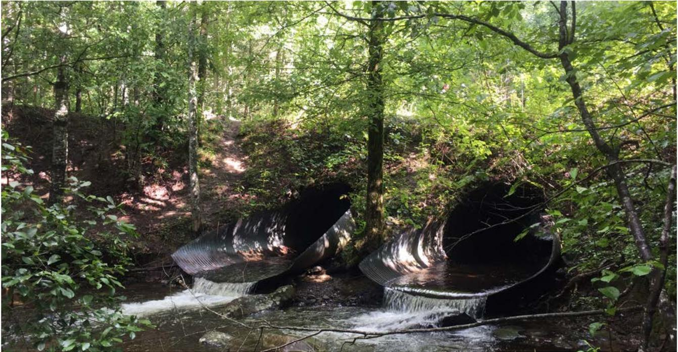
After: This open-bottom, prefabricated arch culvert replaced the failed Mill Creek stream crossing in 2019. Credit: Katie Owns/TNC
