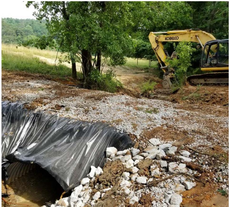
**After:** Newly installed 8-foot culvert allows aquatic and terrestrial passage (fencing to exclude livestock was added later). Credit: Vance Crain/SARP
