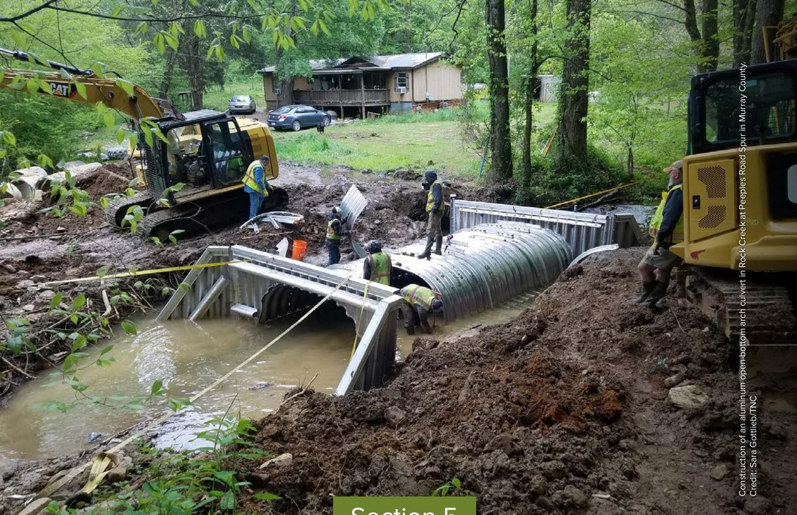
Construction of an aluminum open-bottom arch culvert in Rock Creek at Peeples Road Spur in Murray County.
